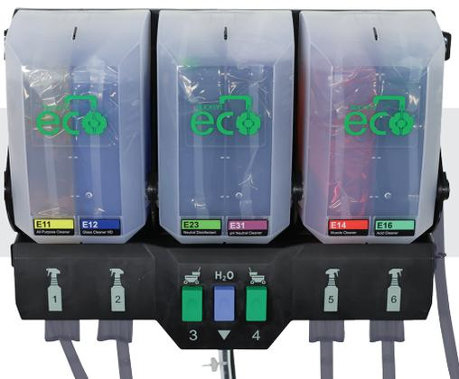
Chesapeake is now testing the Eco® Proportioning Program for use in their weight rooms and HPAC building. Eco proportioning systems automatically dilute concentrated products accurately, saving time and money.
